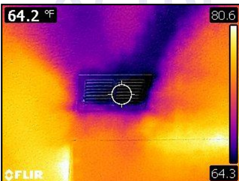
Air conditioning functional, temperature 64 degrees
