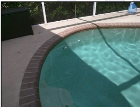
Pool light functioning
