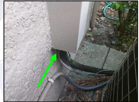
Spray foam shroud shut
